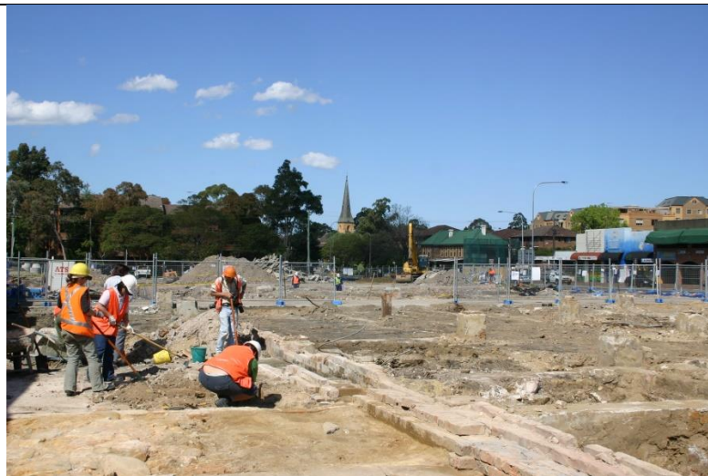
Figure 3.23 Commencement of clean up following removal of slabs and fills Area A-B. Looking East IMG_598 September 2006
