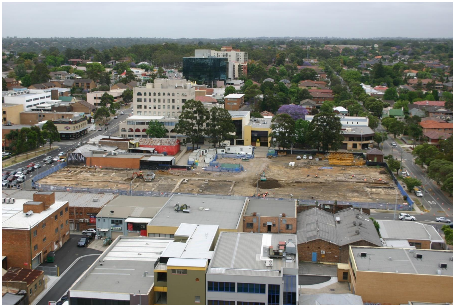
Figure 1.3 Study Site During Excavations Looking South. AMAC Group, 26 th October 2006, IMG_976
